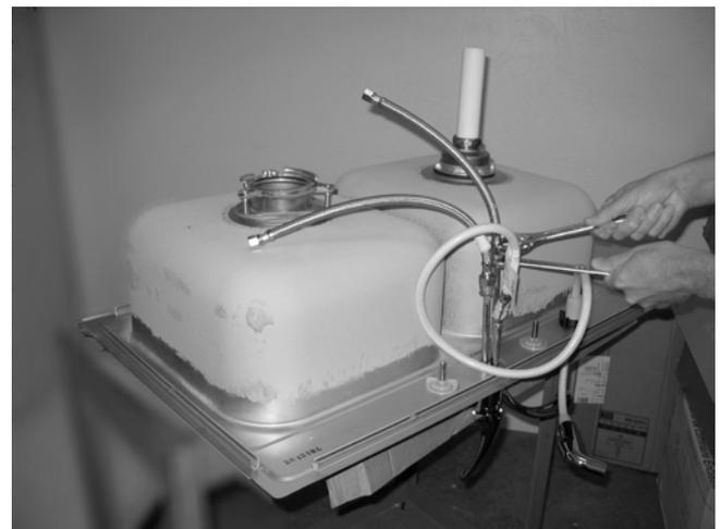
3. Connect the continuous waste assembly to the strainers. If you're installing a food disposal, this step will have to wait until the sink is mounted in the countertop. But if you just have 2 strainers, it's easier to assemble the drainage plumbing interconnecting the two bowls before the sink is installed in the countertop.
