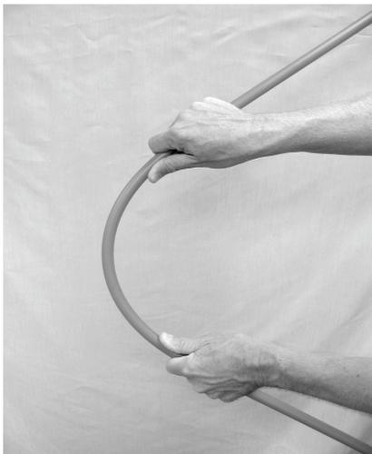
PEX can be bent into a fairly tight radius, but bend no tighter than a radius 6 times the outer diameter of the pipe.
